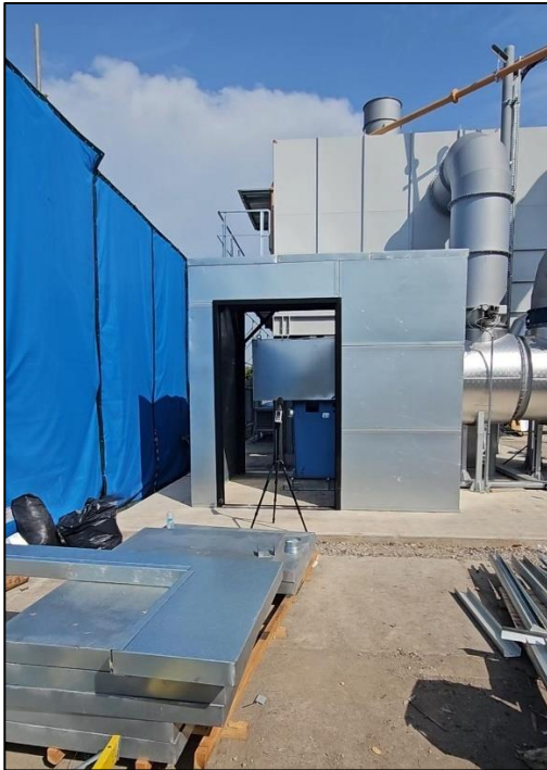
Fig 8a – Regenerative Thermal Oxidiser (RTO) Motor/Fan in Housing - 1
