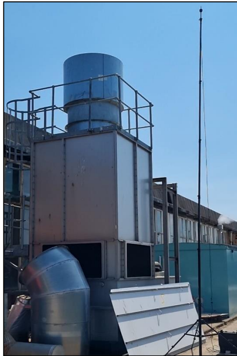
Fig 9 – Water Cooling Tower (Canal-Facing)
