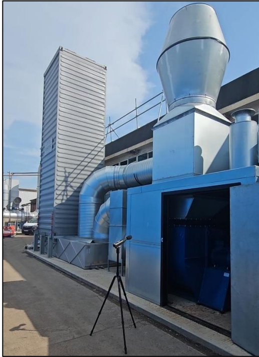
Fig 14 – Carbon Filter
